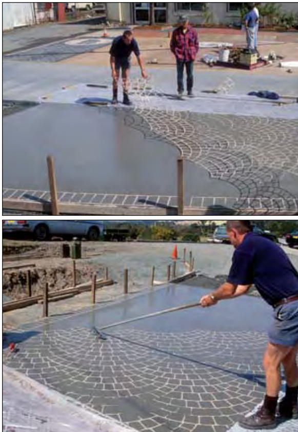
Figure 9.9 Placing and embedding the stencil into the 'wet' concrete
