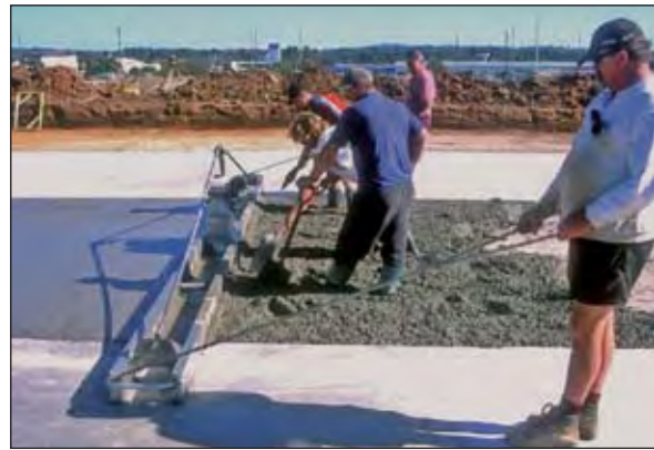
Figure 4.6 Use of a vibrating screed
