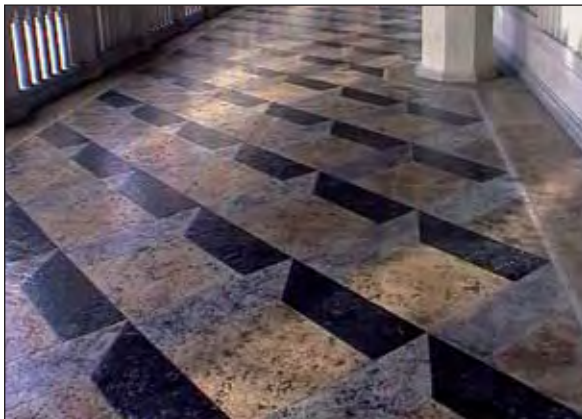
Figure 9.3 Chemical stains used to create patterns
