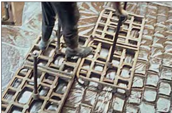
Figure 9.14 Stamping concrete – slate and cobblestone textures
