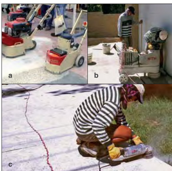
Figure 9.20 Methods of honing concrete surfaces. (a) Dry process, (b) wet process and (c) hand tools for edges
