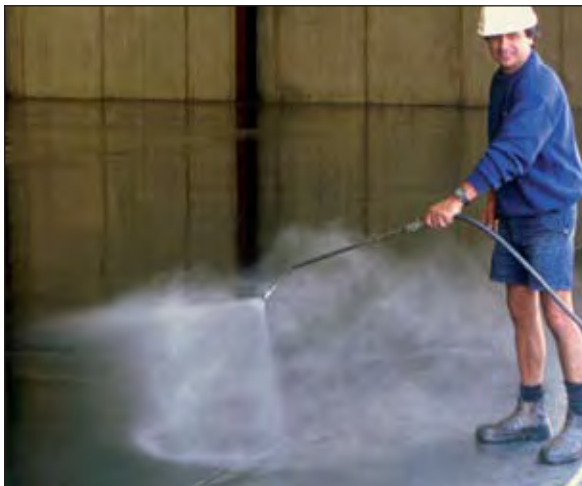
Figure 4.12 Spraying on a curing compound
