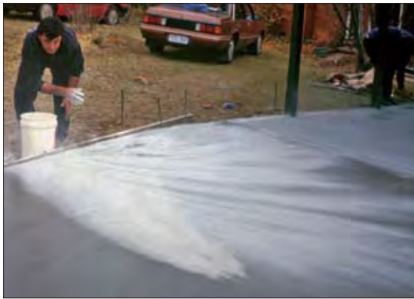
Figure 9.13 Applying release agent
