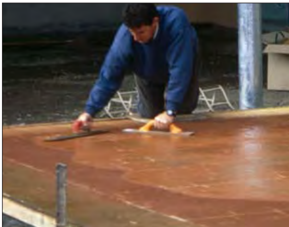
Figure 4.10 Hand trowelling with steel trowel
