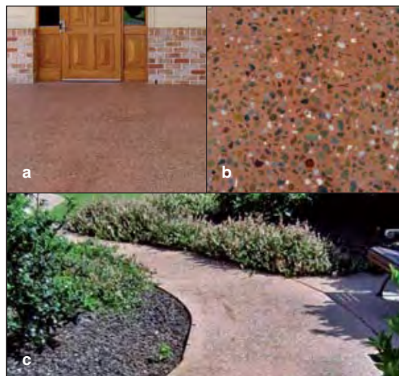
Figure 21 Examples of honed finishes. (a) Patio slab, (b) honed finish at 80 to 100 grit and (c) path
