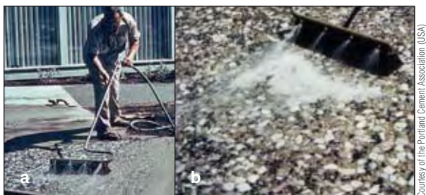
Figure 9.17 Washing off the surface cement mortar (a) to expose the aggregate (b)
