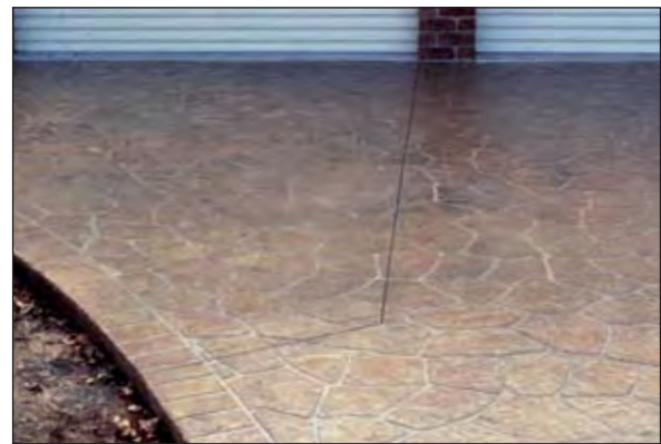
Figure 6.14 Joint perpendicular to slab edge
