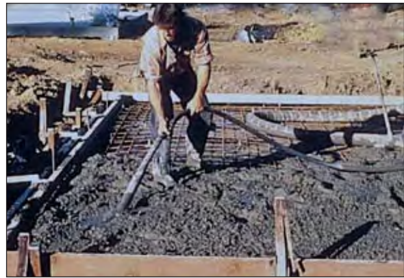
Figure 4.4 Use of immersion (poker) vibrator
