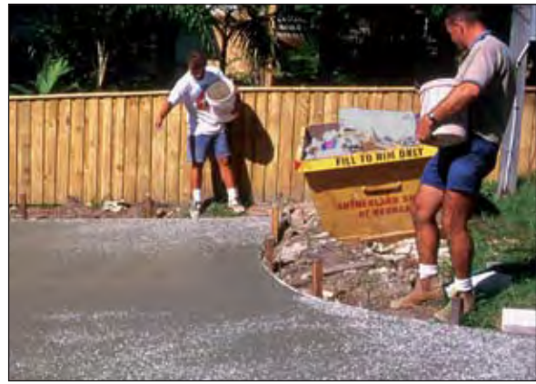
Figure 9.16 Seeding the concrete surface with selected aggregates
