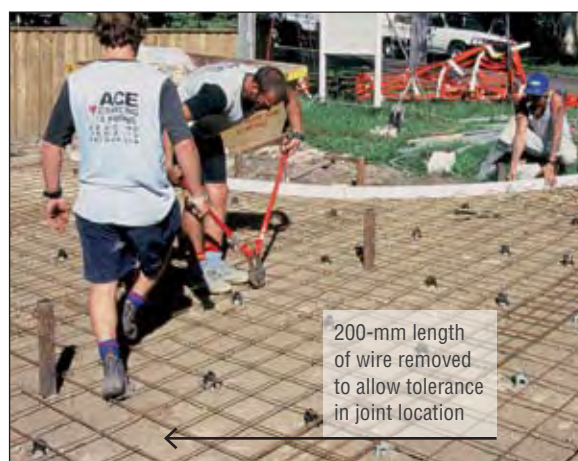
Figure 6.12 Reinforcement fixed in position and mesh being cut at control joint locations
