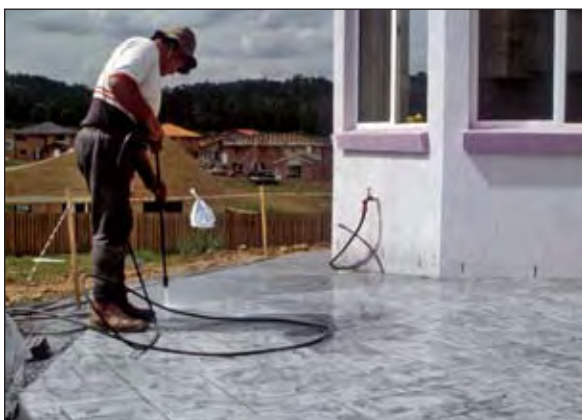
Figure 9.15 Removing the release agent
