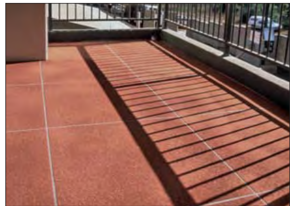
Figure 9.23 Spray-on topping with stencilled pattern
