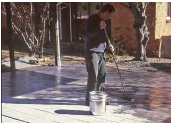
Figure 9.12 Sealing the surface
