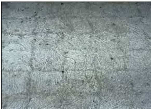
Figure 6.4 Plastic settlement cracks above mesh
