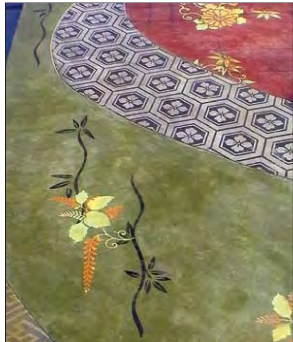
Figure 9.5 Dyes and tints produce strong vibrant colours not possible with stains – red, yellow and orange. Chemical stain used for mottled green background and patterned border.
