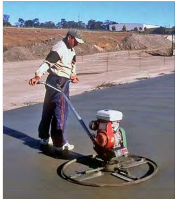
Figure 4.11 Trowelling by machine
