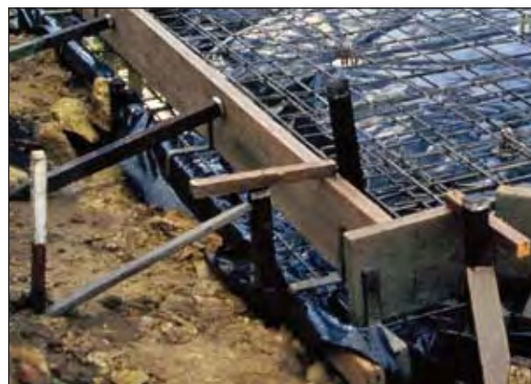
Figure 5.5 Edge rebate formwork with brackets and edge board
