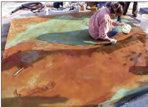
Figure 9.4 Chemical stains can pond on flat surfaces to allow good penetration
