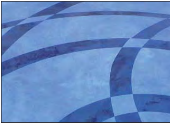
Figure 9.6 Dark blue areas are a coloured cement-based micro-topping approximately 1 mm thick trowelled onto the surface. Light blue colour is from dye washed over the surface.
