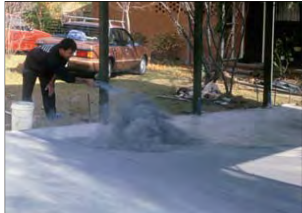
Figure 9.1 Dry-shake topping being applied
