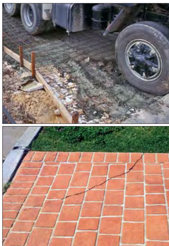
Figure 8.3 Poor subgrade may cause cracking of pavement
