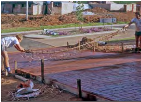
Figure 9.10 A stencil being removed
