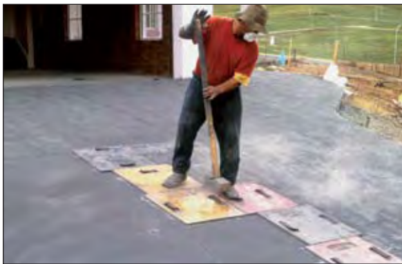
Figure 9.13 Applying release agent
