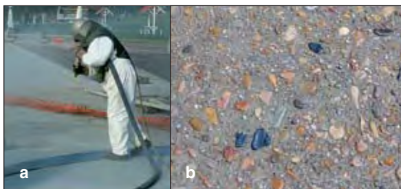
Figure 9.18 (a) Abrasive blasting and (b) close-up of finish
