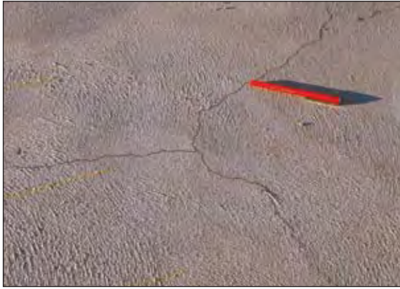
Figure 6.1 Plastic shrinkage cracking
